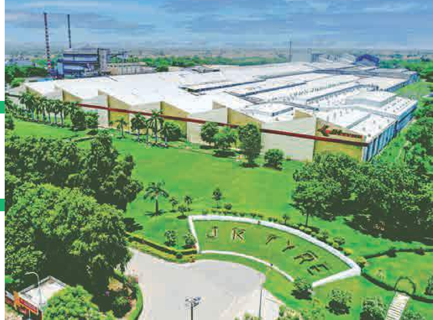
JK Tyre Plant, Banmore, Gwalior
