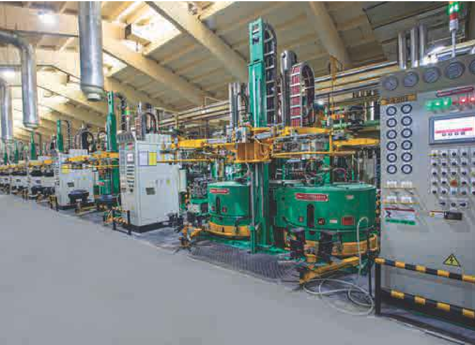
JK Tyre Plant, Banmore
